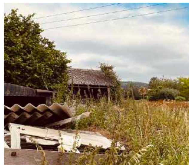
Existing stable building in the centre of the site
