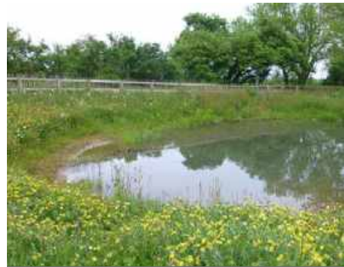
Overground attenuation pond
