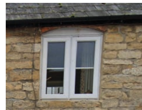
Window close to eaves
