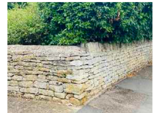
Stone boundary wall with hedge planting
