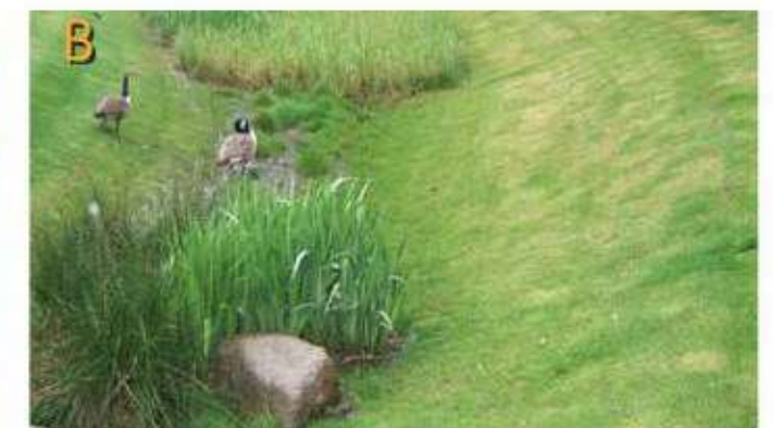
Incorporate swales within the open space and along woodland belts, softened with shrub and riparian planting.
