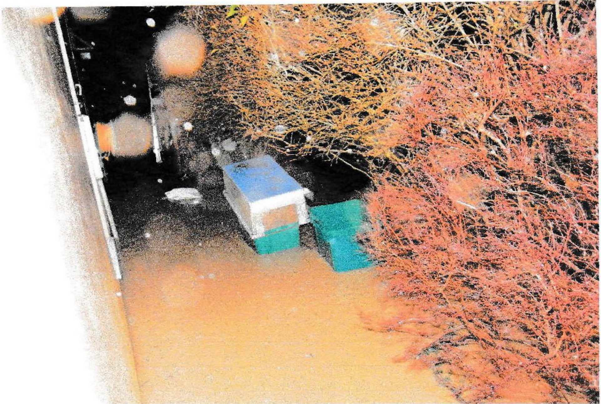
2 Orchard Road, water at 6pm overflowing from culvert over the ground alongside the house. 23.12.2020
