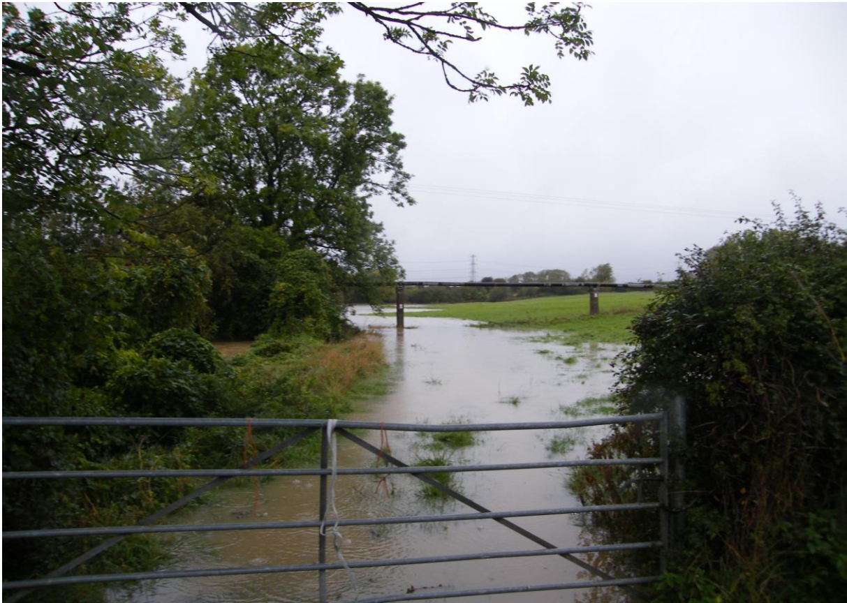
View from Arch Bridge looking west (taken 3 and 4 October 2020)
