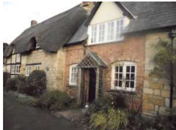
Fig. 29 View of Grade 2 listed cottages in Church Road
